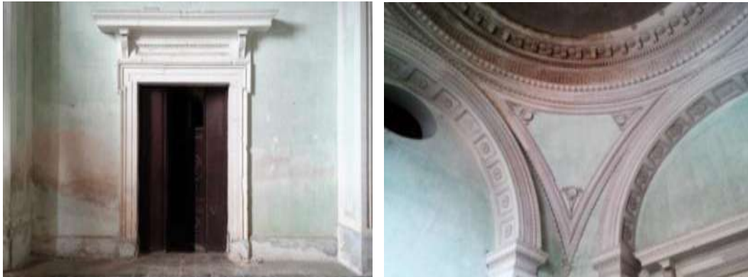
Details of the simple Neoclassic architecture and of the chapel's interior decoration.
