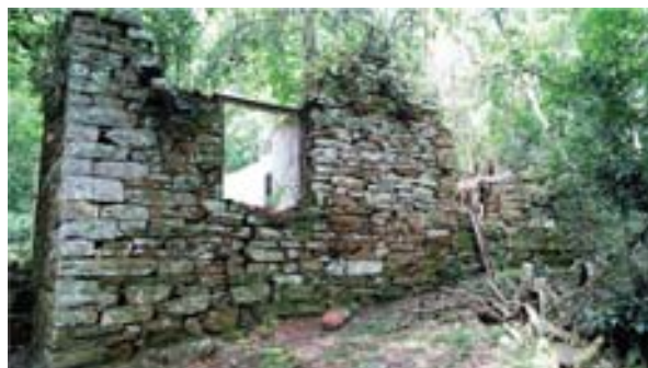
Fig. 1 Lateral wall of Structure I. Notice the use of almost uncut stone and the modern machine-made window
